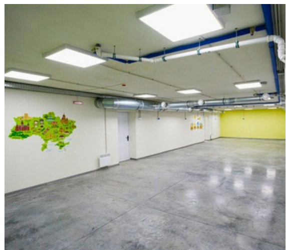
Completed School Bomb Shelter Renovation
