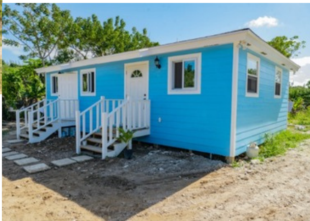
Before and After GER 3 Home Repairs
